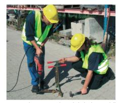
For pavers that are extremely interlocked, a hammer drill can be used on the AHW to save time and money. The extraction foot lever AHW is equipped with a wire brush for cleaning the profiled spring steel blades after each extraction. Using this will help provide maximum grip on each paver.
