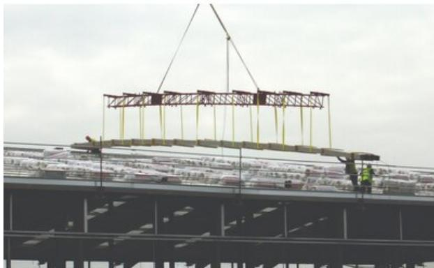
Our Roof Sheet Beams are a lightweight modular spreader beam suitable for long, light loads and have been specially developed to suit roofing sheets.
