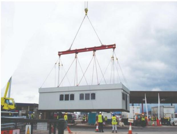
Multipoint Lifting Beams have lifting points at various intervals along the bottom. Ideal for lifting fragile but heavy items that require lifting on several point.
